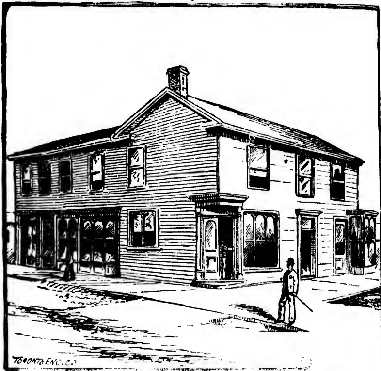
THE OLD CAVAN ARMS—NORTH-WEST CORNER ADELAIDE AND VICTORIA STREETS
